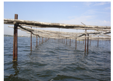
ZOOM ON A SHELLFISH REARING TABLE, FRANCE. IT IS MADE OF RAILS OF SEVERAL METERS DRIVEN IN THE GROUND ON WHICH HORIZONTAL WOODEN OR METALLIC POSTS ARE FIXED. THE REARING ROPES ARE THEN SUSPENDED TO THESE POSTS. SOURCE: THIERRY LAUGIER.
